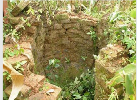
Figure 35. Updraft kiln constructed of bricks
