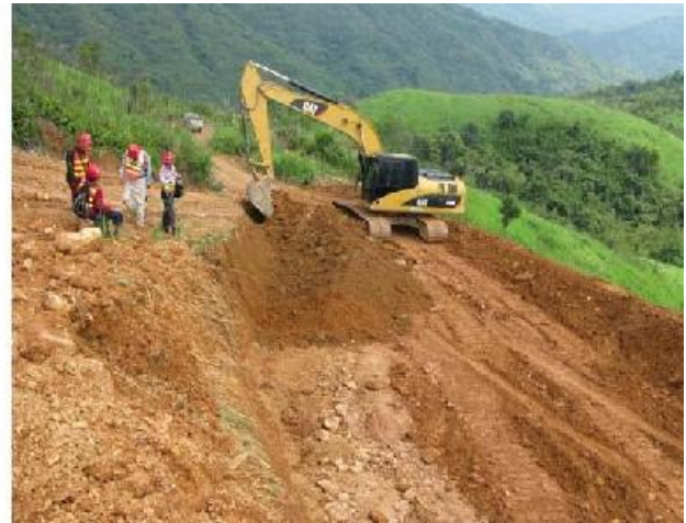
Dam Site: Road quarry to Bridge #1, Road slope improvement at curve sta.0+300 (May 2011)
