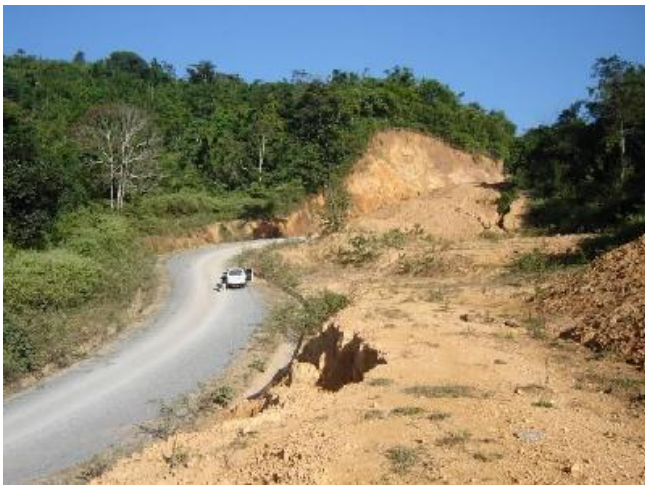
Slope failure along access road, crushed stone pavement
