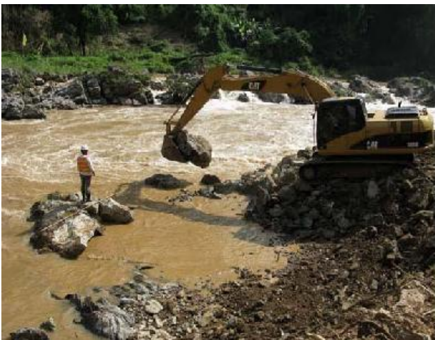
Dam Site: Temporary cofferdam construction for pier no.#2 of Bridge #1 (May 2011)
