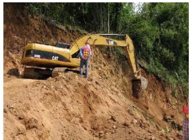
Dam Site: Road quarry to Bridge #1 Road widening and slope improvement (May 2011)
