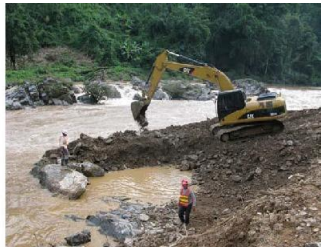
Dam Site: Temporary cofferdam construction for pier no.#2 of Bridge #1 (May 2011)
