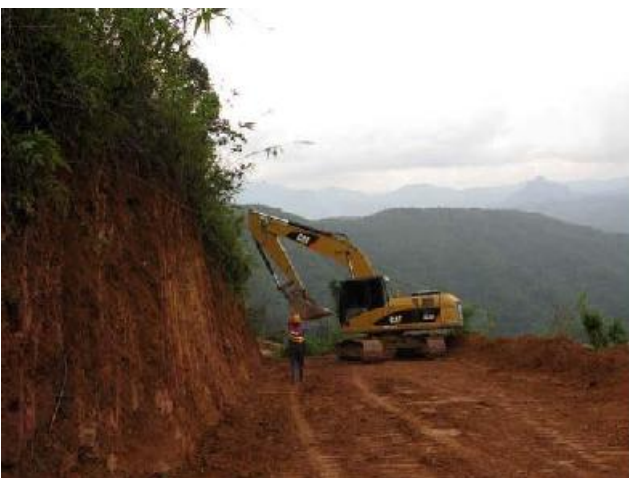
Dam Site: Road quarry to Bridge #1, road widening from sta. 0+000 to 0+200 (May 2011)
