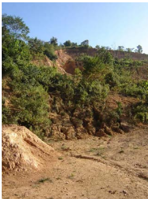
Slope failure and natural re-vegetation at former borrow site
