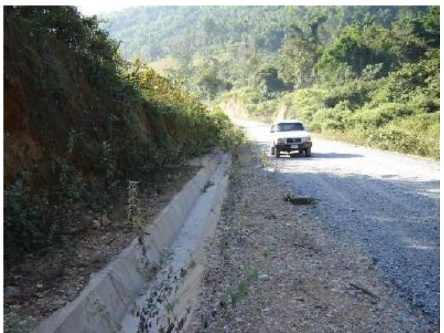
Side drains and crushed stone pavement of access road
